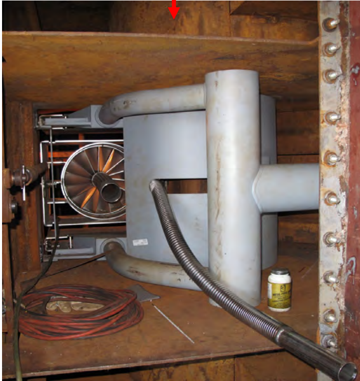
T-Fired Burner Components (Rear)
