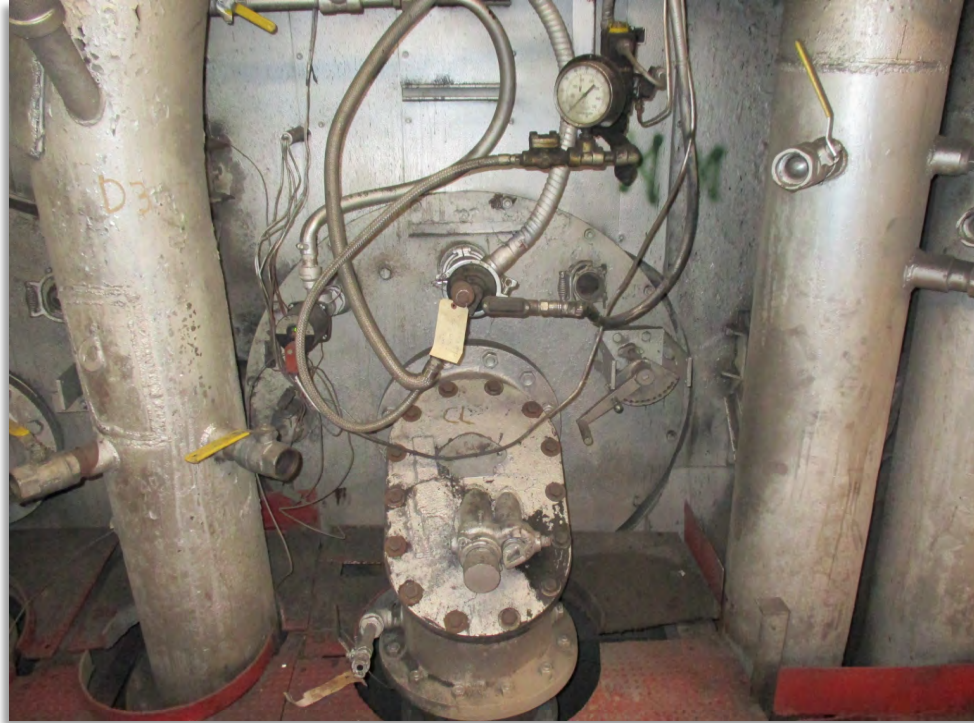
Existing Coal Burner
